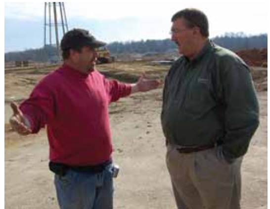
While waiting for the trucks to arrive Cospers discusses a job with paving foreman Todd Hemphill.
